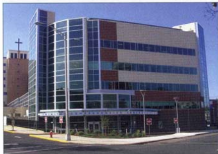
The Tinitas Comprehensive Cancer Center was recently honored as "Project of the Year" by the Metro NY/NJ Chapter of the Construction Management Association of America.
